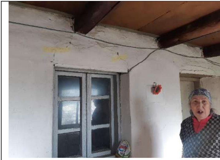
Crack markers in the houses of vil. Tskere
