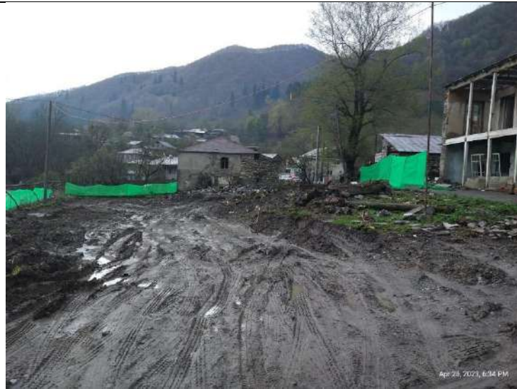
Fenced off site after demolishing the house in village Arakhveti
