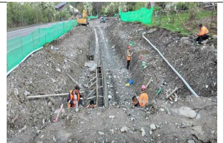
Installation of temporary sewage pipe for villagers of Arakhveti
