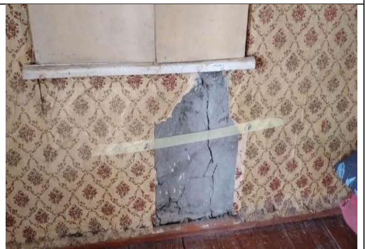
The crack on local resident's house marked at the pre-construction phase, village Tskere, 14.03.23
