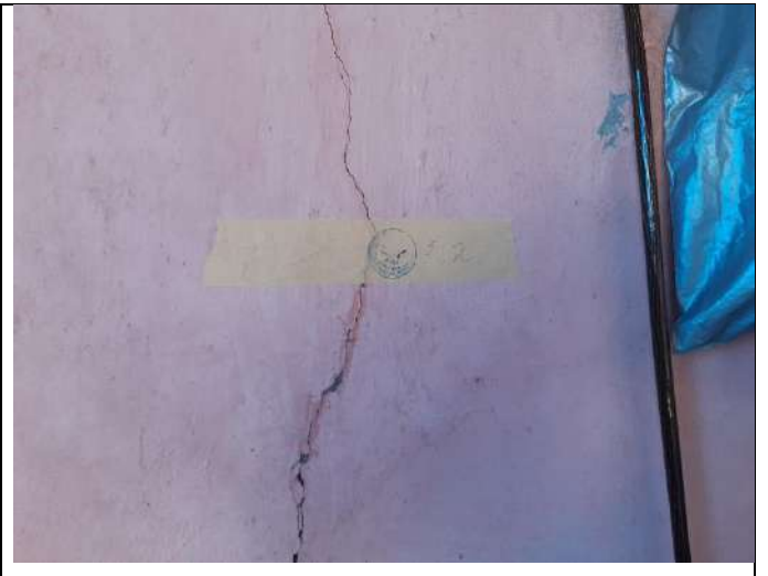
Crack markers in the houses of vil. Tskere
